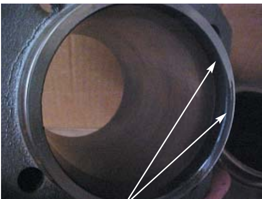
Fig. 5.1.5 Irregular seat between the upper cylinder liner part and the cylinder head
